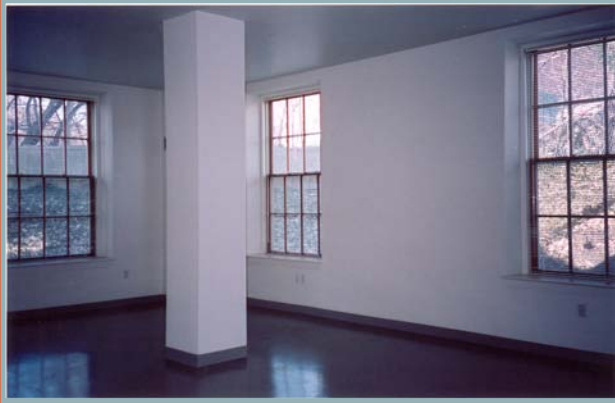
One of the finished units inside the Walter Baker building.
