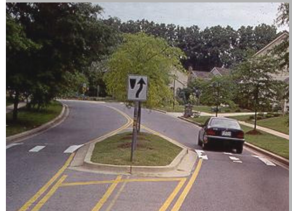
A combination of speed humps and a median island forces this car to slow down in a residential area. Source: http://www.trafficcalming.org .
