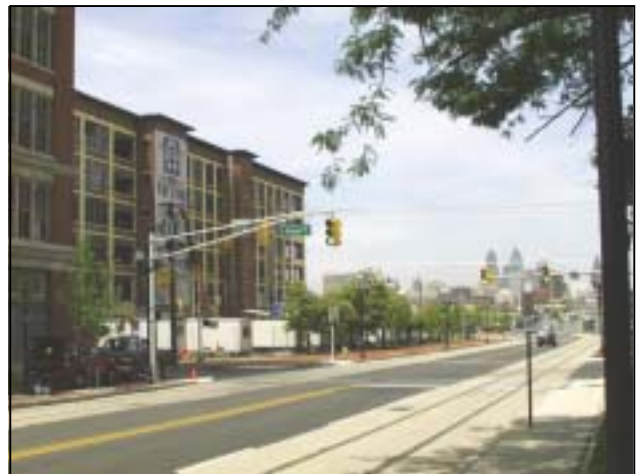
From left to right, the southbound platform on Cooper Street, testing an LRT vehicle on Cooper Street, and the Victor Building redevelopment project.
