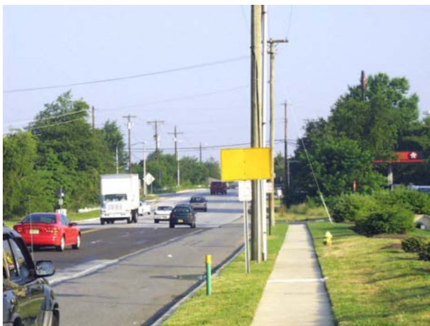
Replace existing faded warning sign (Right Lane for Exit Only) on westbound Center Square Road approaching I-295 interchange
