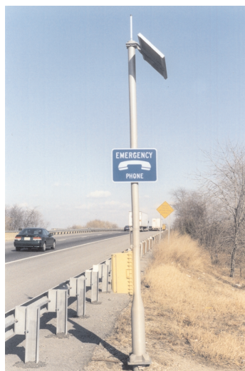
Self-efficient, solar powered emergency call box on I-295
