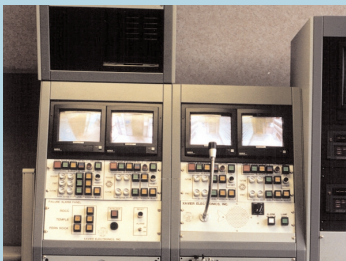
Closed circuit television monitors at SEPTA's Transit Operations Center
