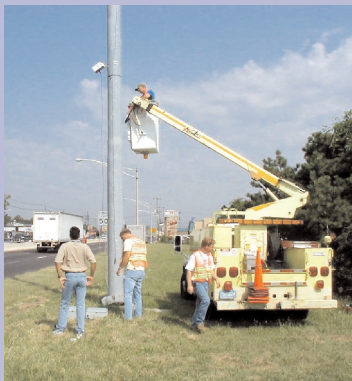
NJDOT, Cross County Connection TMA, L-3 Communications and Rutgers University have formed a partnership in a demo project to install roadway sensors that will collect congestion information and disseminate it to travelers via pagers. This photo shows sensors being installed at the intersection of I-295 and NJ 73 in Mount Laurel.
