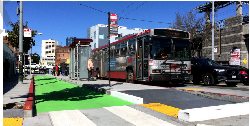
Below: A floating boarding island functions similarly to a trackless trolley curb extension, but accommodates a curbside bicycle lane. Source: San Francisco Bicycle Coalition
