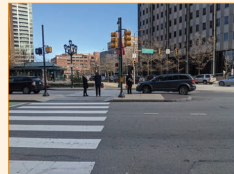
A pedestrian island provides a safe space for pedestrians to wait if the crossing distance is too long. Source: DVRPC
