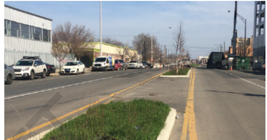
Above: A raised median with green stormwater infrastructure on North American Street in Philadelphia. Source: DVRPC.
