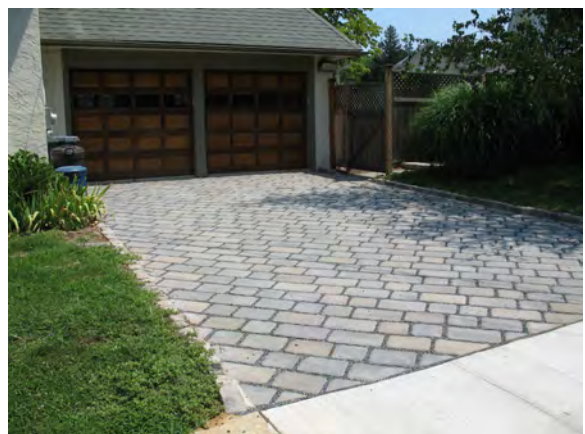
Phil Witmer’s porous driveway surface.
