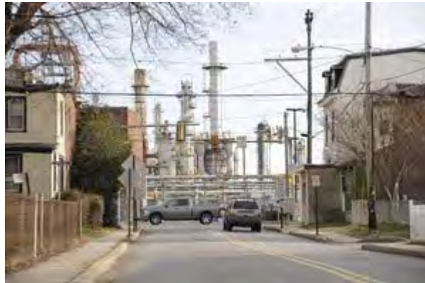
The main gate to the ConocoPhillips refinery in Trainer, Delaware County, is at Main Street and Post Street. CLEM MURRAY / Staff Photographer
