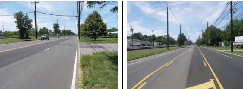
A road diet was implemented along River Road in Cinnaminson, New Jersey. The image on the left shows the roadway before the conversion. The image on the right shows the roadway after the road diet, in which a center turn lane was created. SOURCE: DVRPC
