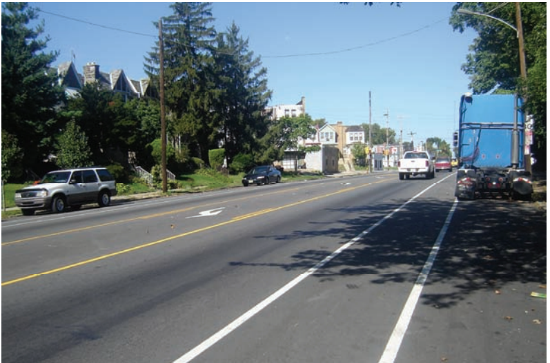
A road diet project on Stenton Road in Philadelphia consisted of a two-way center left-turn lane, one travel lane in each direction, and bike lanes in each direction. Curbside parking along the roadway was retained. SOURCE: DVRPC
