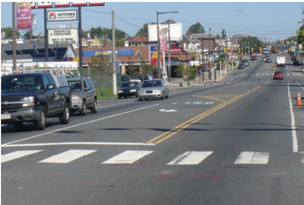
A road diet conversion for Ogontz Avenue in Philadelphia was completed in 2003. SOURCE: DVRPC
