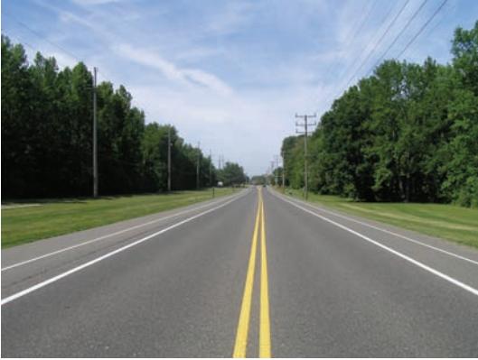
A road diet project on Fort Dix Road in Pemberton, New Jersey added shoulders and bike lanes. SOURCE: DVRPC
