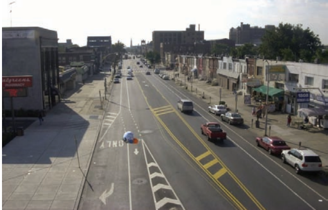
Philadelphia's Allegheny Avenue was reconfigured through a road diet. At the top is the roadway prior to the road diet. Below is the roadway after the road diet, with pedestrian pockets, a turning lane, and a bike lane. SOURCE: John Boyle, Greater Philadelphia Bicycle Coalition
