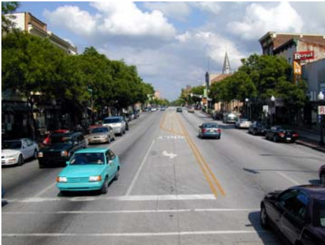
High Street BEFORE Improvements
