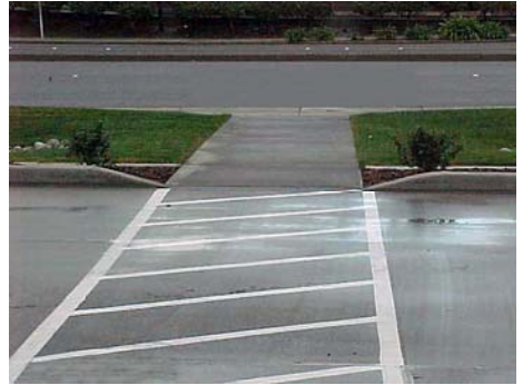
Pedestrian walkway over grassy swale with culvert for stormwater runoff.
