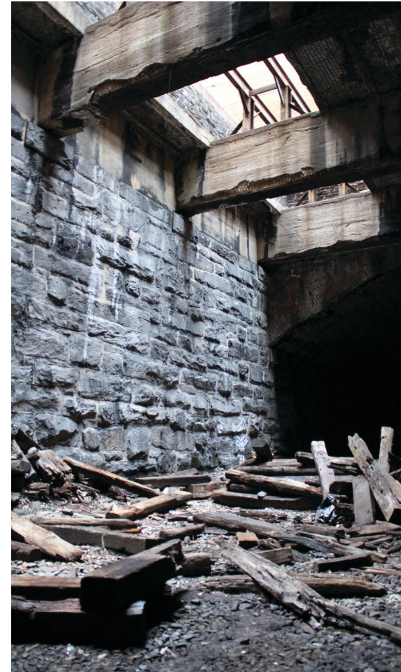
Figure 23: City Branch Tunnel View
