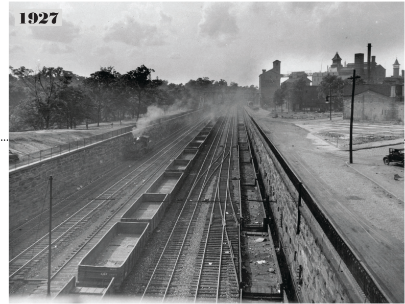
Figure 7: City Branch View From Pennsylvania Avenue & 27 th Street
