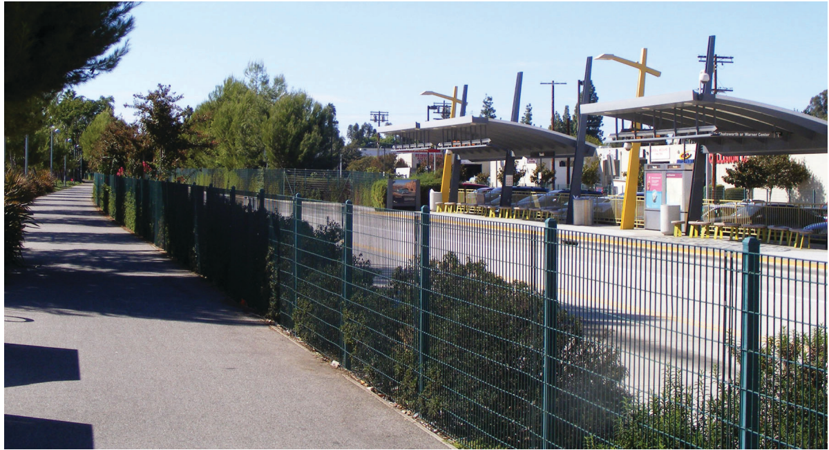
Figure 55 : Reseda Station, Orange Line
