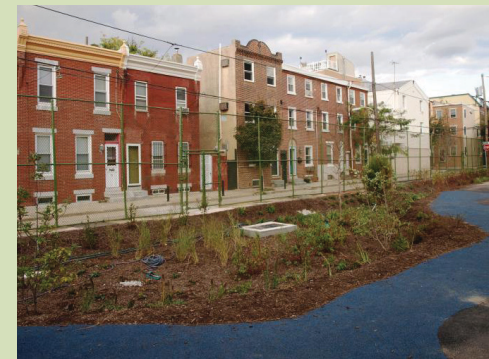
Figure 75: Green Stormwater Infrastructure at Nebringer School in Bella Vista.
