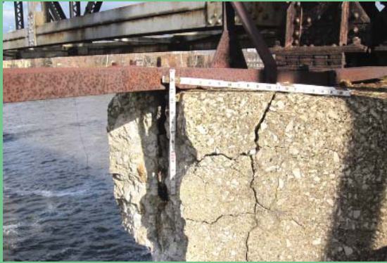
The Norristown High Speed Line Bridge over the Schuylkill River is more than 100 years old and is substantially corroded. While the high and medium scenarios envision replacing this bridge in the next five years, the low would defer its replacement to somewhere in the 2020s, risking the chance of service disruption on this line.
