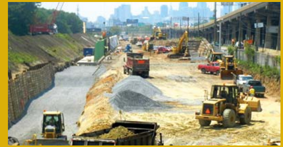
Richmond Street in Philadelphia is being widened and relocated to help handle additional traffic during I-95 viaduct reconstruction. Traffic management during major reconstruction projects increases costs, but is necessary to keep traffic moving.
