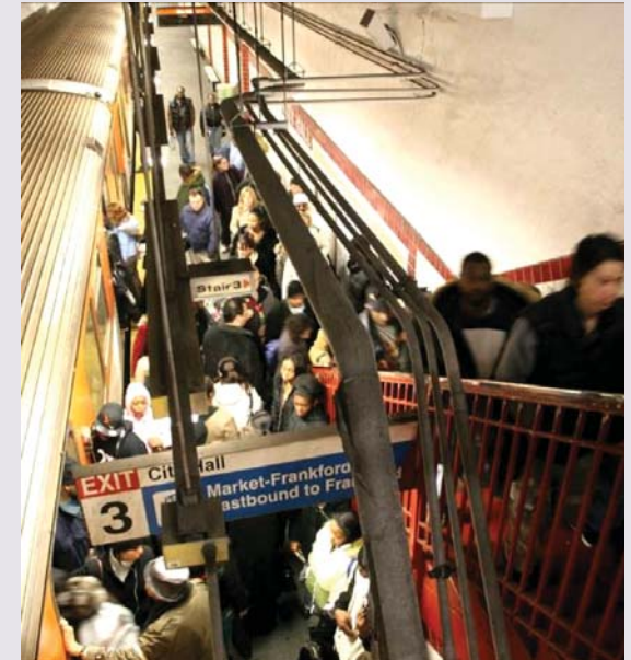
Philadelphia's City Hall Station has not undergone a major renovation since it began service in 1928. The station suffers from water damage, corrosion, and concrete spalling. The station platforms and stairways are too narrow to deal with the crush of peak-hour use, and the station lacks elevators and other important Americans with Disabilities Act accessibility features.
