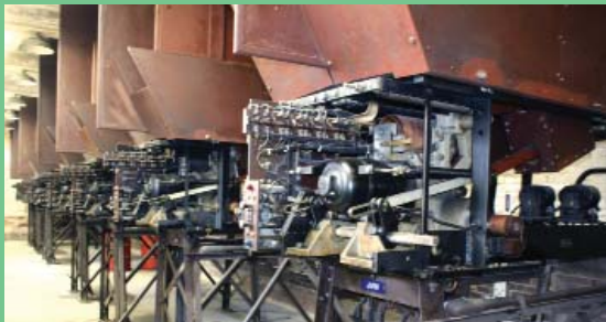
The Jenkintown Substation was constructed in 1930. It supplies power to the Lansdale-Doylestown, Warminster, and West Trenton regional rail lines. This is one of 15 regional substations that are past their useful life.
