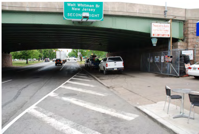
Figure 8: Freeway Underpasses along the Sidepath
