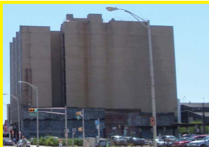
Photo 10: Site 7 (Source: DVRPC, 2010)
