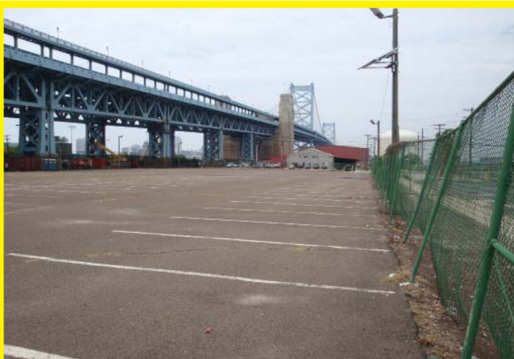
Photo 4: Site 1 (Source: DVRPC, 2011)
