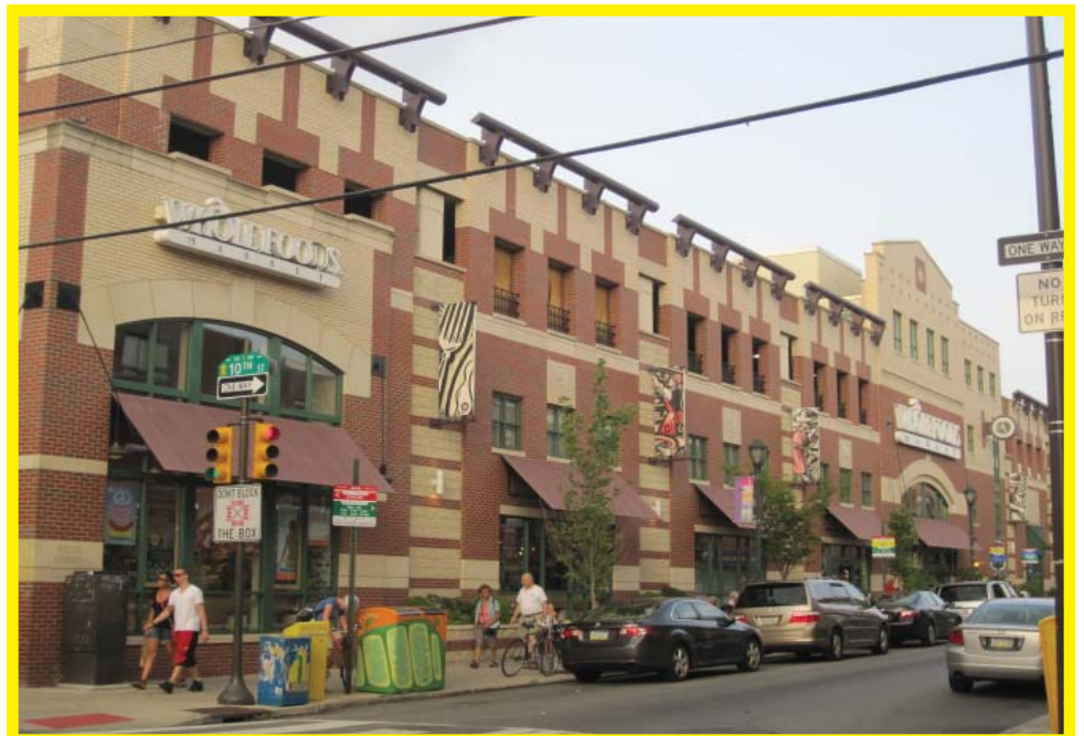
Photo 14: Philadelphia Whole Foods Mixed-Use Parking Structure (Source: DVRPC, 2011)
