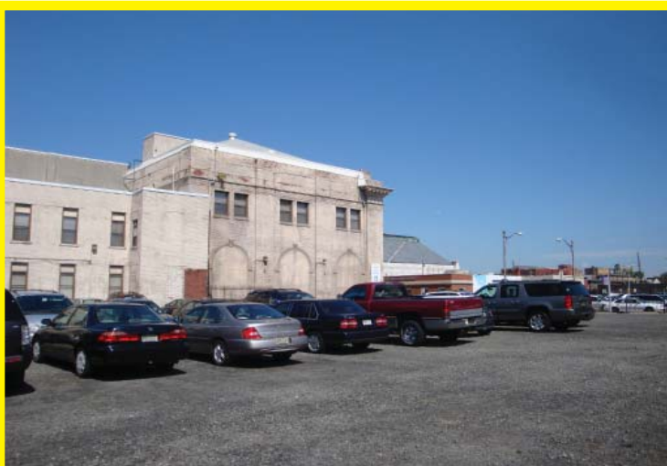
Photo 8: Site 5 (Source: DVRPC, 2010)
