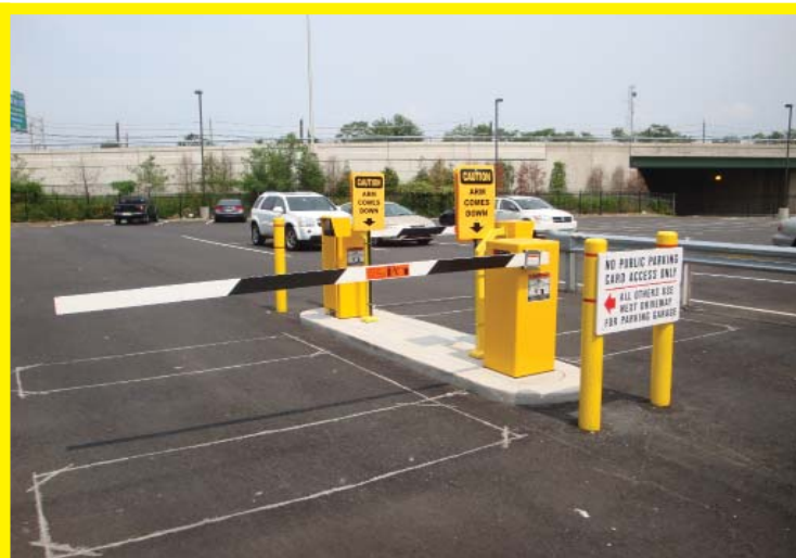
Photo 12: Site 9 (Source: DVRPC, 2010)
