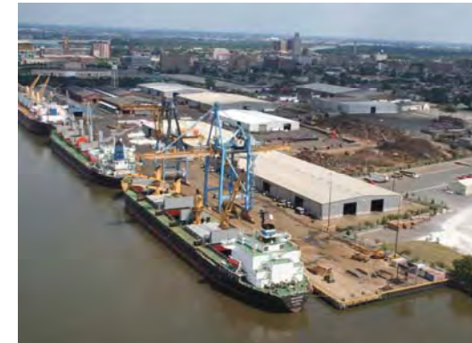
Beckett Street Terminal in Camden County, New Jersey. Source South Jersey Port Corporation
