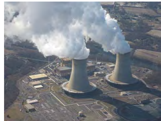
Limerick Nuclear Generation Station in Montgomery County, Pennsylvania. Source Wikipedia
