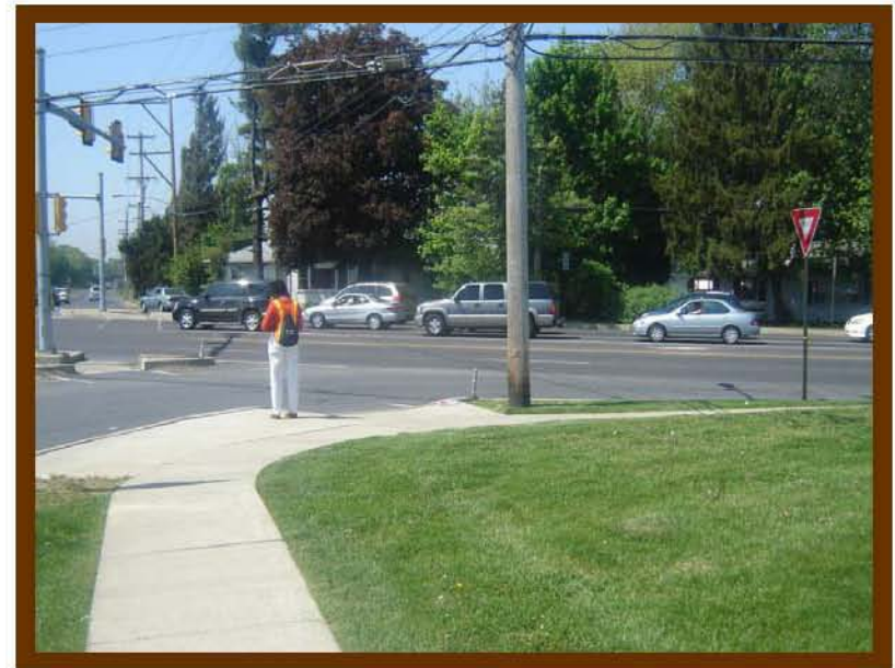
Faded pavement markings and "yield" sign at the channelized right turn beyond the crosswalk at northwest corner of the Knights Road intersection
