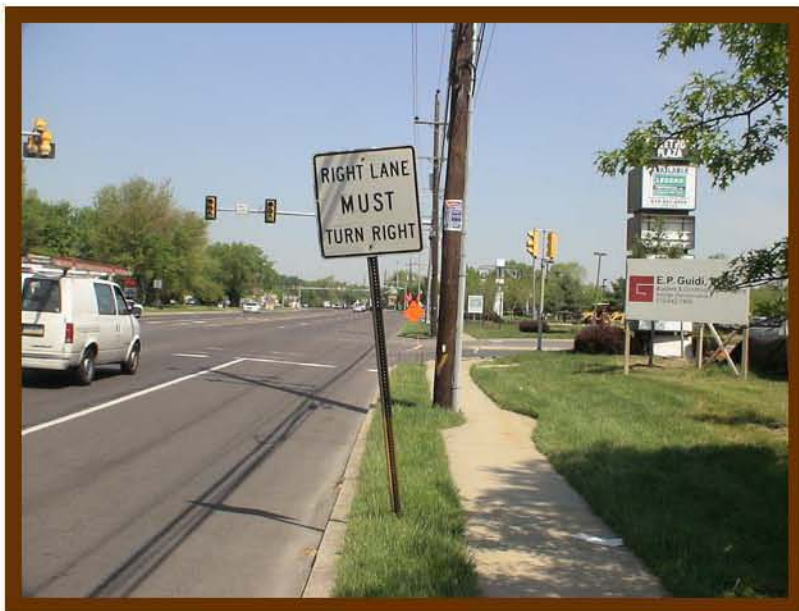
Sign leaning into the travelway
