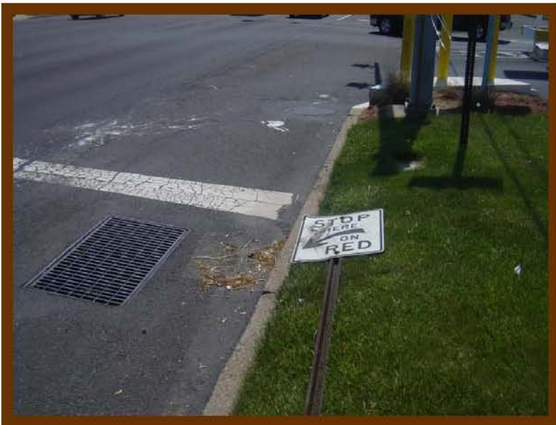
Sign knocked down at entrance to Bensalem Plaza
