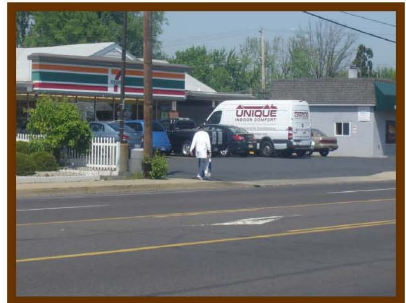
Turn arrow pavement marking is faded
