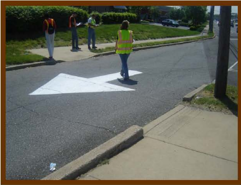
Street Road entrance to Kohl's – large oversized arrow and no pedestrian crosswalk
