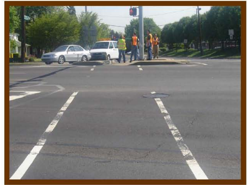
Pavement markings faded, typical throughout the corridor
