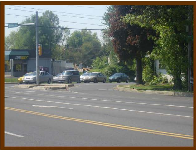
Faded pavement markings and no "yield" sign at the channelized right turn at the Knights Road intersection
