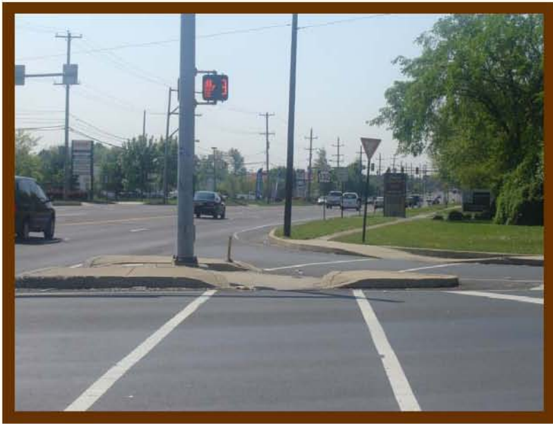
Yield sign beyond pedestrian crosswalk—typical in the corridor
