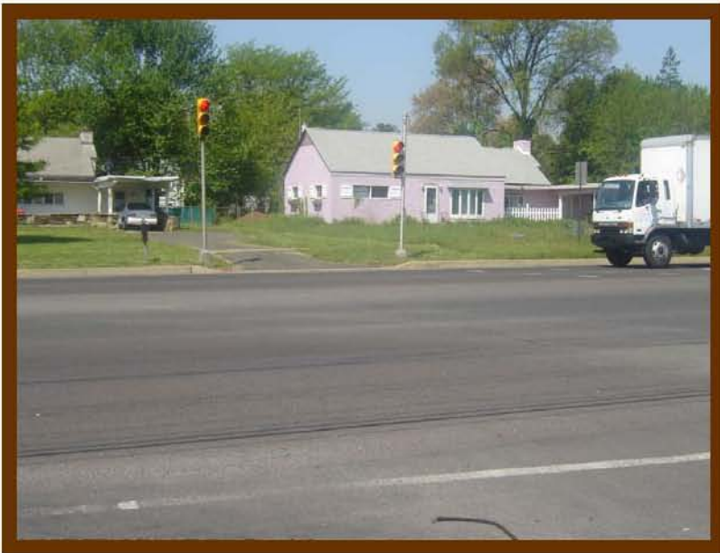
Two traffic signals facing the shopping center driveway west of Castle Drive
