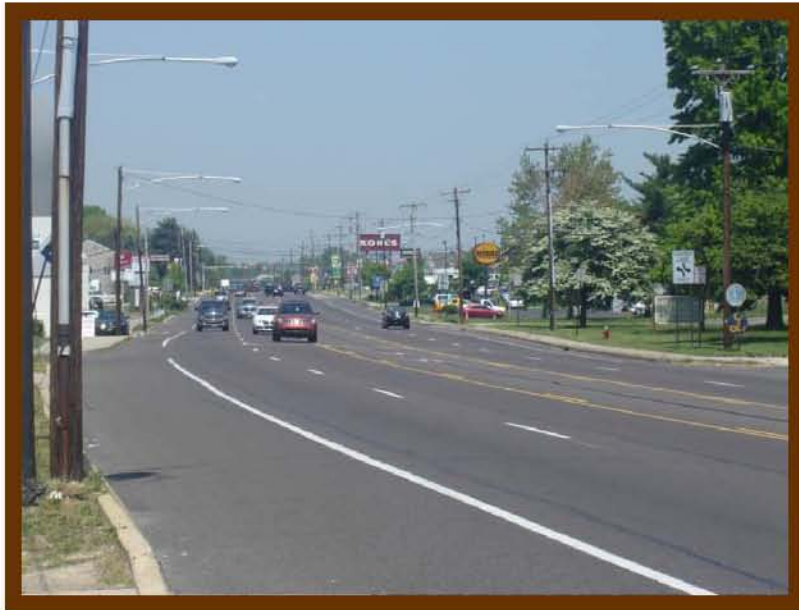
Curb cuts along Street Road
