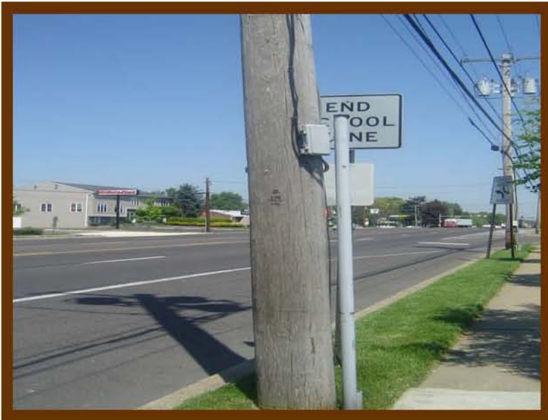
Sign blocked by utility pole and sign in the background twisted
