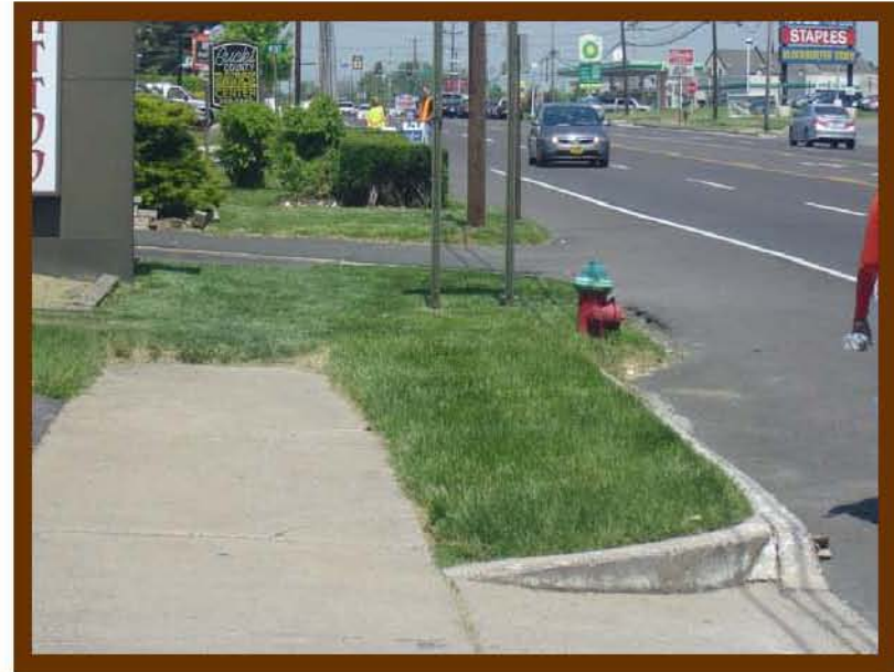
Sidewalk abruptly ends
