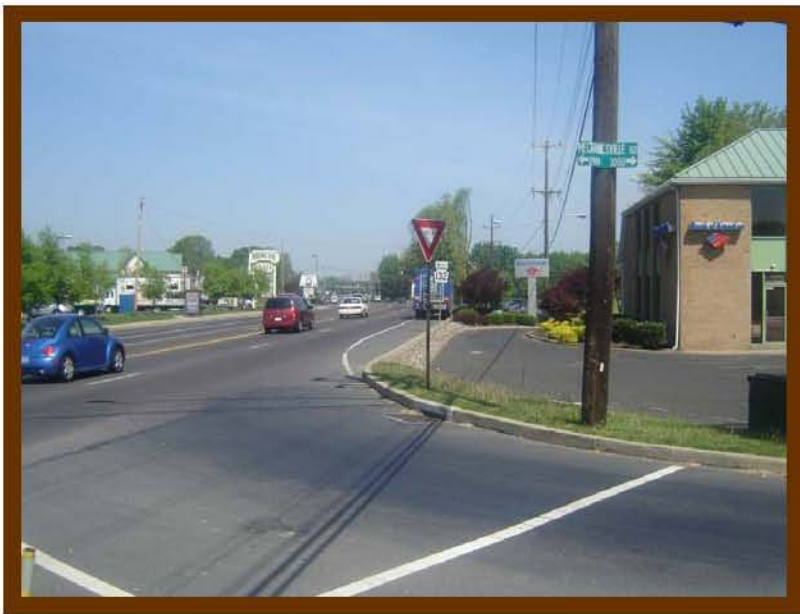
West of Mechanicsville Road there are no sidewalks; there are no curb ramps at the crosswalk
