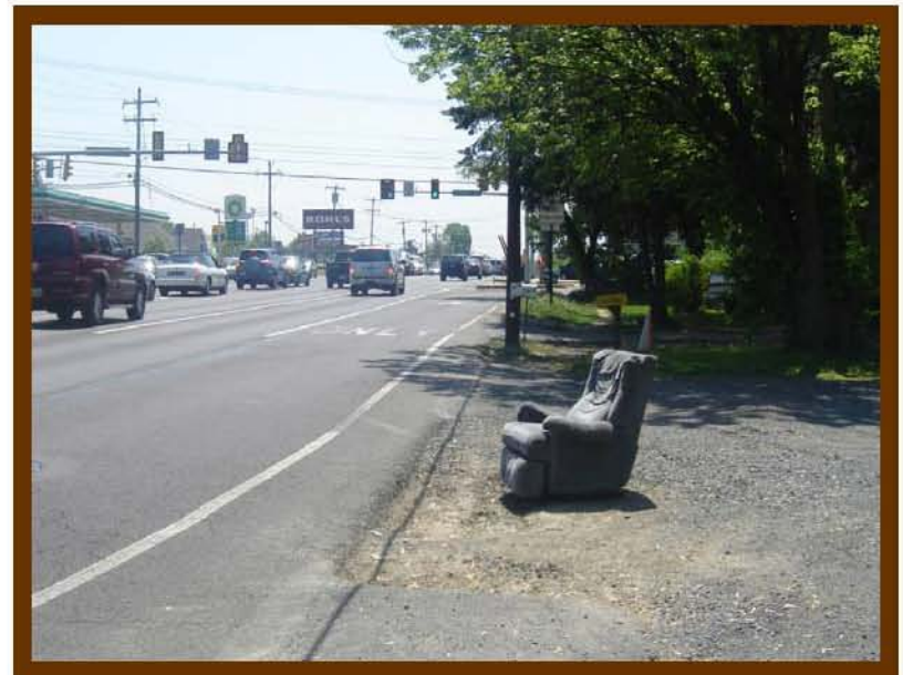
No sidewalk and undefined driveway on Street Road
