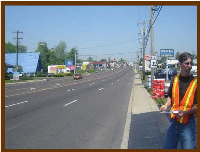
Curb cuts along Street Road and road configuration
