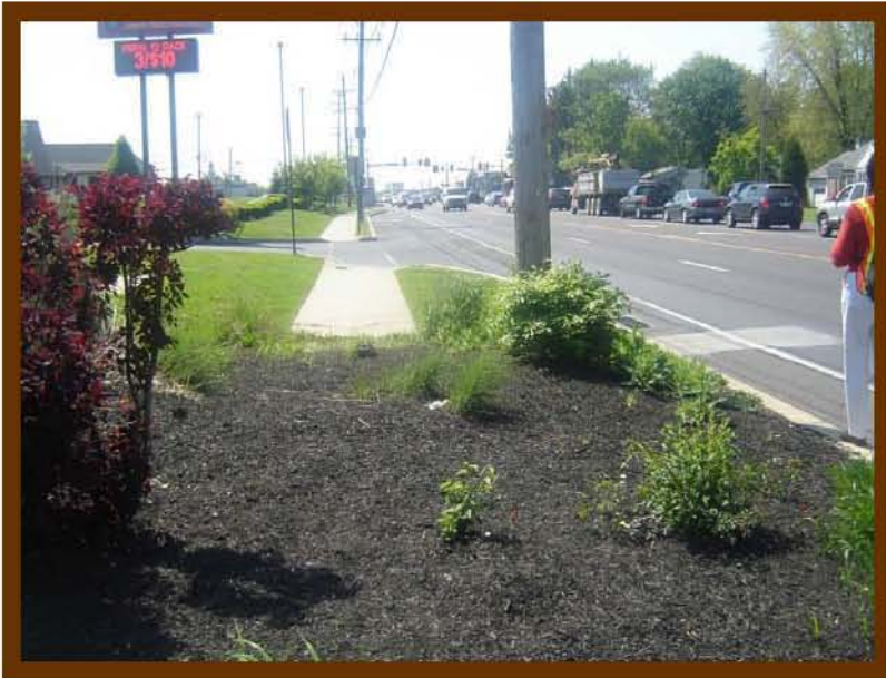
Sidewalk ends abruptly
