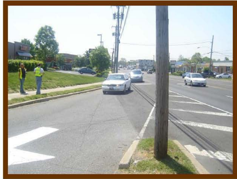
Street Road entrance to Kohl's – geometry allows speeding into the entrance from the main road
