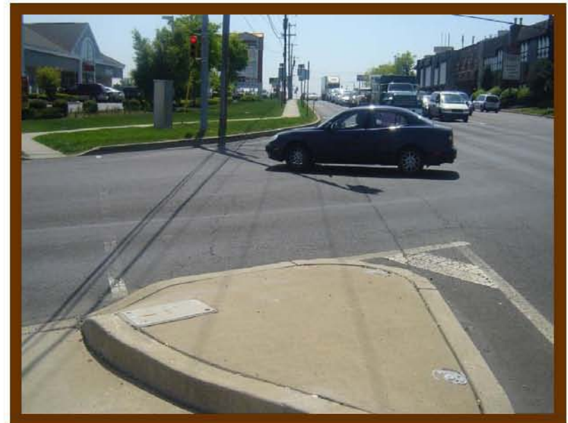
Missing delineators on the channelized island at the Hulmeville Road intersection
