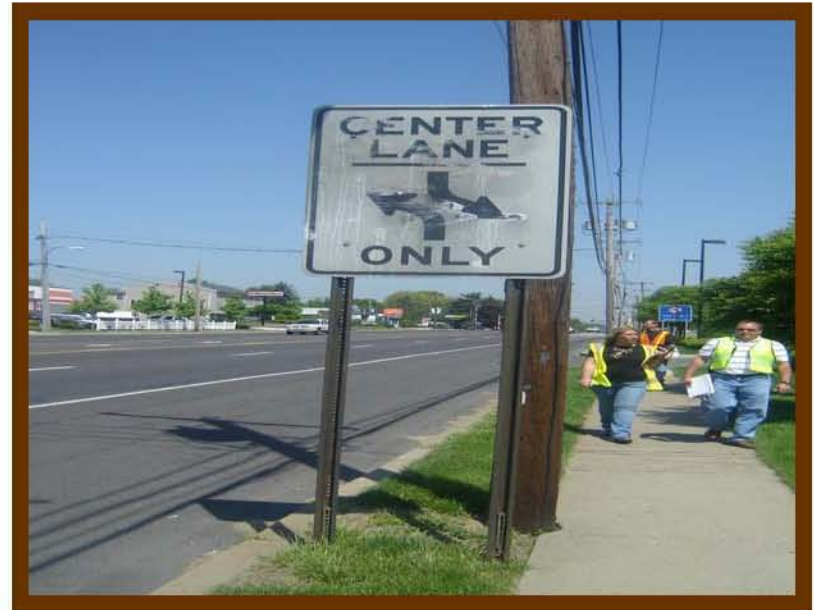
Sign defaced; needs to be replaced
