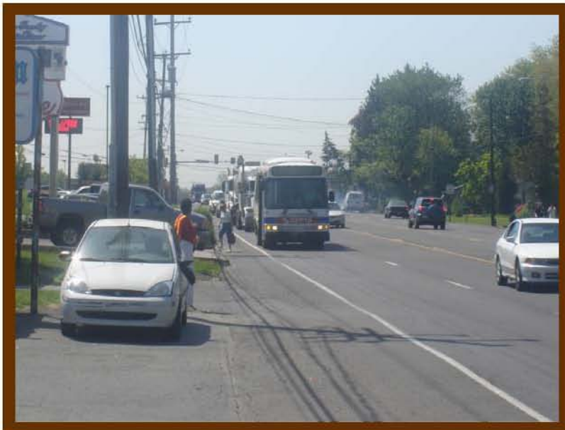
Bus in travel lane dropping of passengers into area with no sidewalks on Street Road, west of Knights Road
