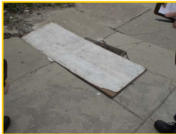
Sidewalk disrepair along Erie Avenue
