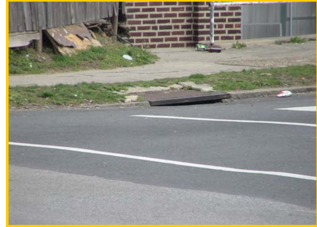
Drainage inlet along Olney Avenue
