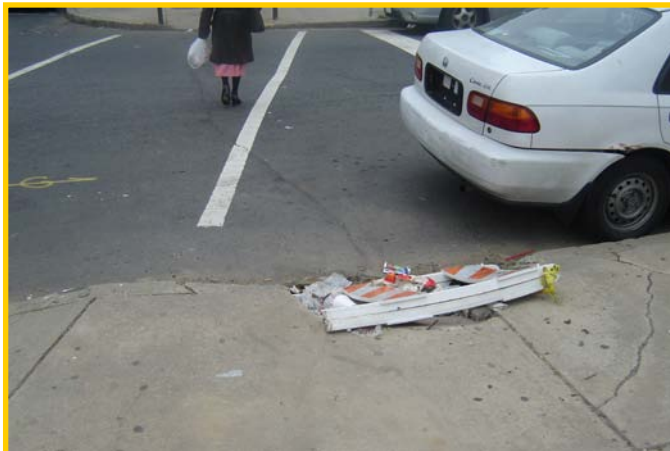
Example of sidewalk disrepair along Erie Avenue, corridorwide issue
