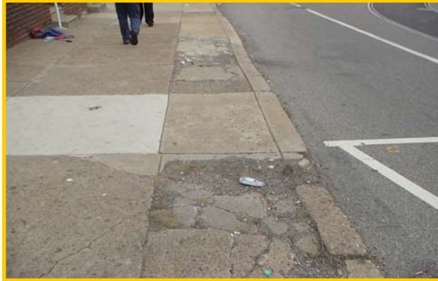
Example of sidewalk disrepair/urban ills, corridor-wide issue
