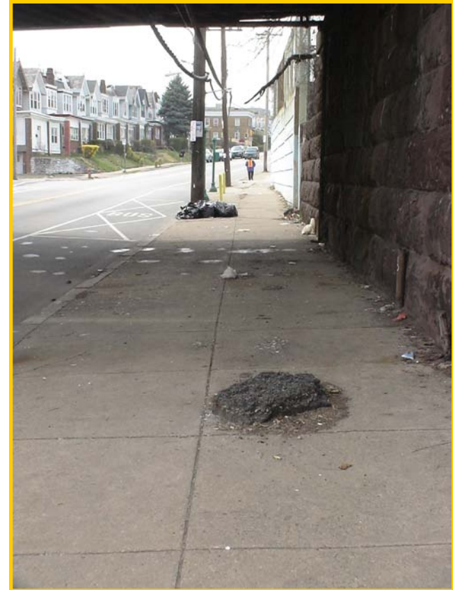
Tripping hazard, general neglect along Olney Avenue
