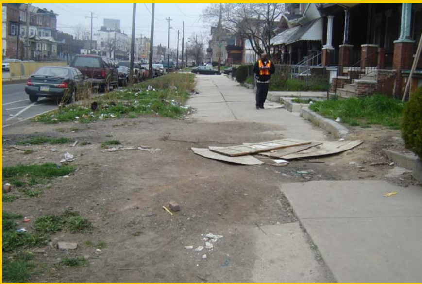
Deteriorated and obstructed sidewalk along Erie Avenue
