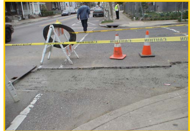
Construction temporarily blocks pedestrian way on Olney Avenue
