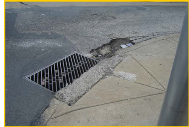
Example of deteriorated infrastructure along Erie Avenue
