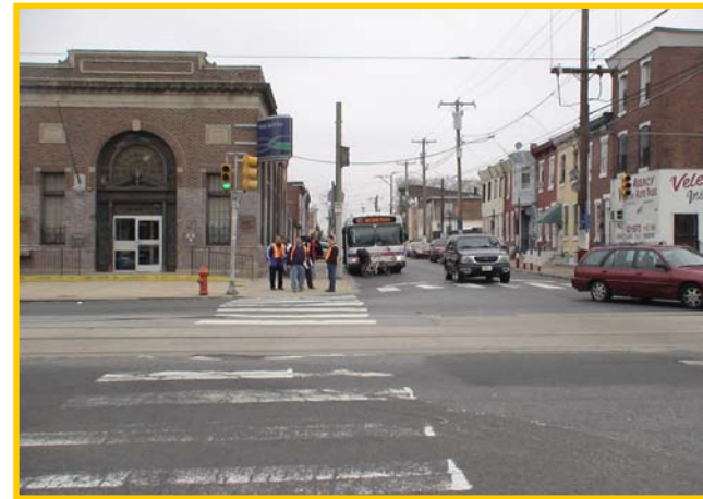
Former trolley right-of-way obstructs pedestrian crossing over Erie Avenue near Rising Sun Avenue, corridorwide issue.
