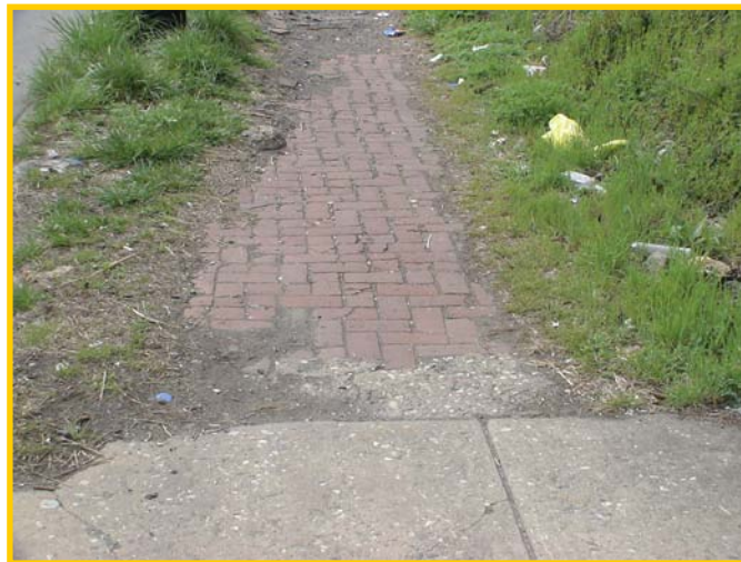
Inconsistent sidewalk type, litter, general neglect
