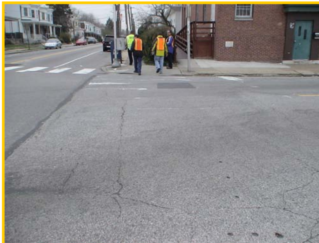
Faded crosswalk over Olney Avenue side street
