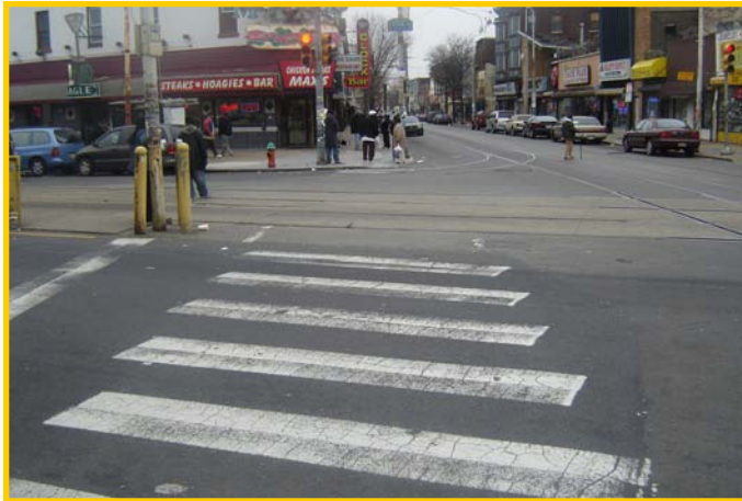
Deteriorated pedestrian crossing near Germantown Avenue
