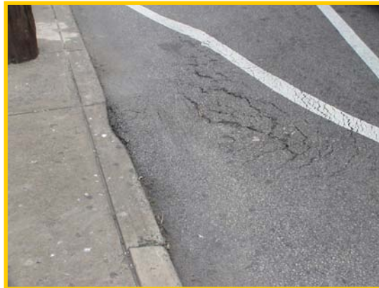
Deteriorated pavement along Olney Avenue
