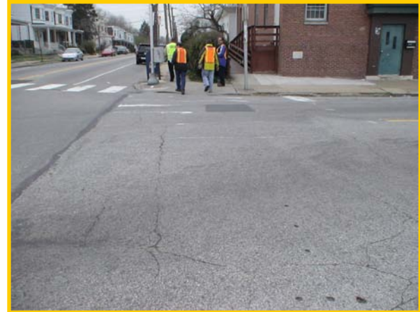
Faded crosswalk markings over side street along Olney Avenue
