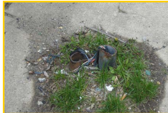
Tripping hazard along Erie Avenue
