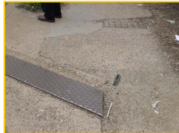
Sidewalk in disrepair between Front and B Streets
