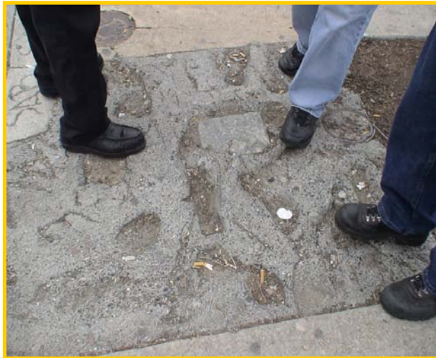
Sidewalk tripping hazard along Olney Avenue near Front Street
