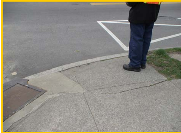
Missing curb ramp along Olney Avenue
