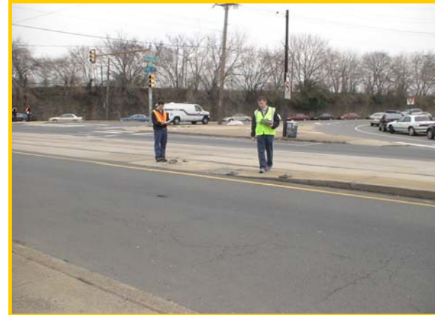
Example of inconsistent center-lane surface treatment at Whitaker Avenue
