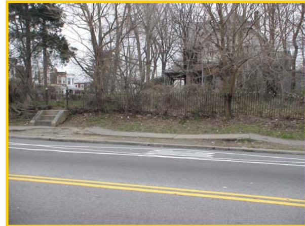
Deteriorated sidewalk at bus stop along Olney Avenue
