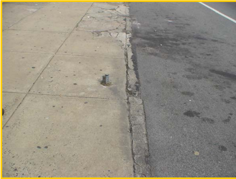
Tripping hazard on Olney Avenue near 10th Street
