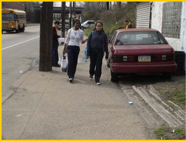
Obstructed sidewalk on Olney Avenue near 7th Street
