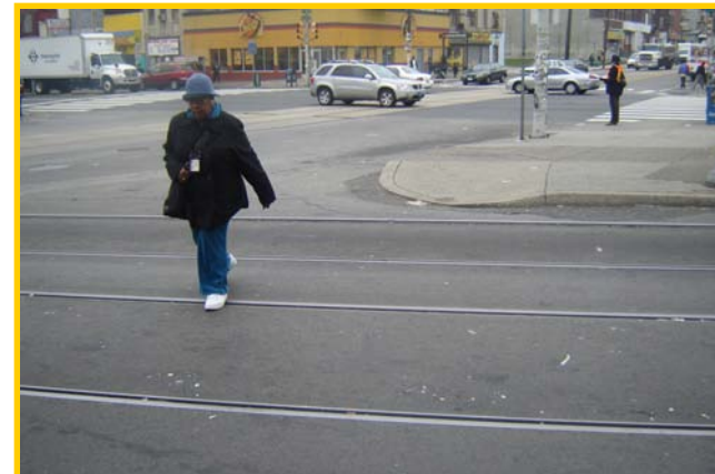
Former trolley tracks create tripping hazard
