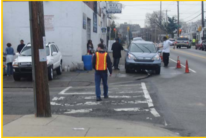
Crosswalk deterioration, sidewalk obstruction at Olney and Fairhill Streets
