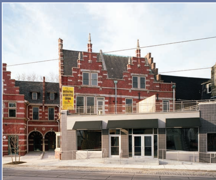
Winston Commons, developed by Mt. Airy, USA contains a mix of retail and condo units. (Source: Mt. Airy USA, photo by Hugh Loomis)
