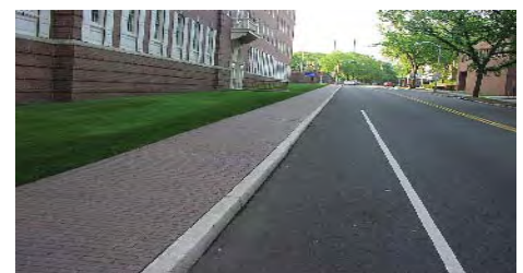
This urban street was retrofitted with a shoulder to enhance bike travel.
