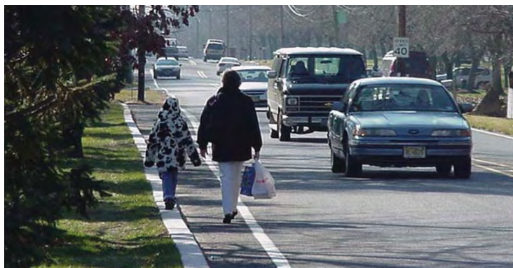
Missing sidewalk links are one of the biggest impediments to pedestrian mobility, particularly in suburban areas in the two states. Pedestrians in these areas must regularly walk in the street.
