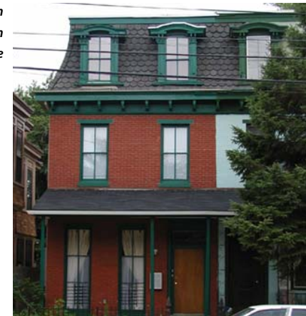
Rehab on Powelton Avenue
