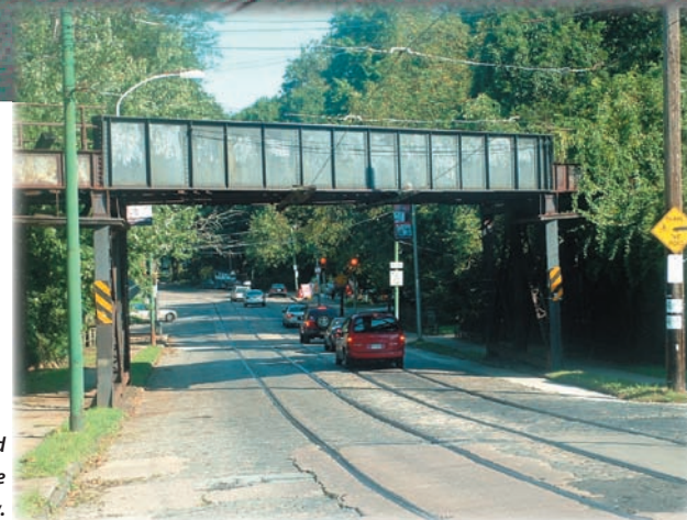
The existing railroad bridge can become a gateway to Mt. Airy.
