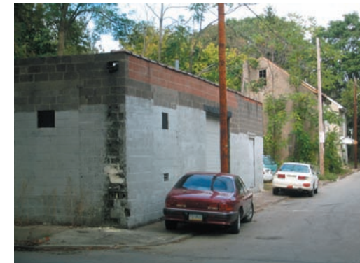
The blank wall of an auto body shop, which is a nuisance use on a residential street.
