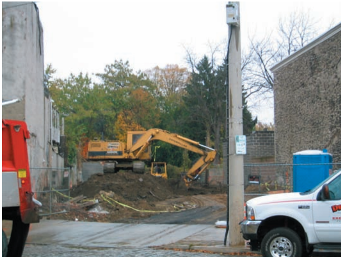
A medical facility is being constructed on the vacant lot that formerly contained two billboards.
