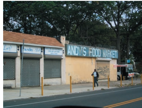
Blank walls have a deteriorating effect on shopping; this store is actually open for business, in spite of its negative appearance.
