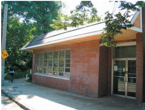
The former Post Office is being redeveloped.
