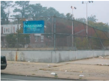
The Pleasant Playground is in disrepair.
