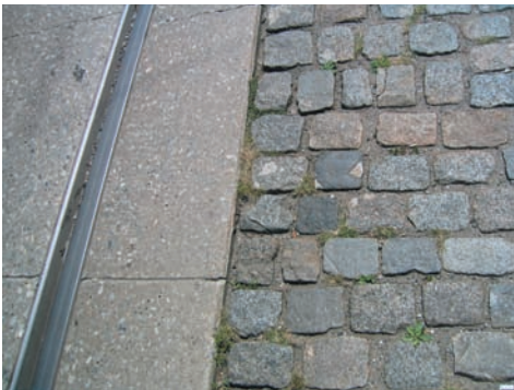
The recently replaced Belgian Blocks of Germantown Ave.
