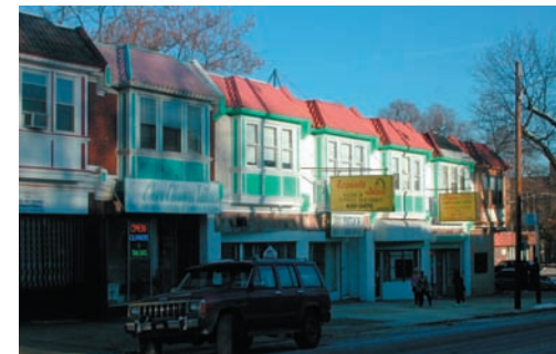
A mixed use building on Chew Ave.
