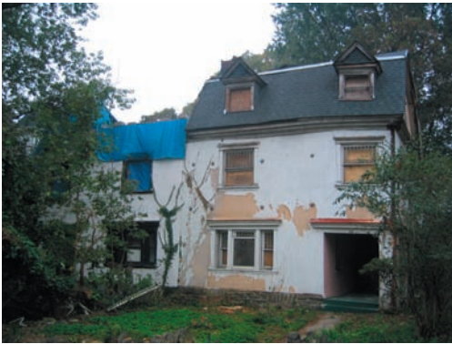
Abandoned house — a deteriorating influence.
