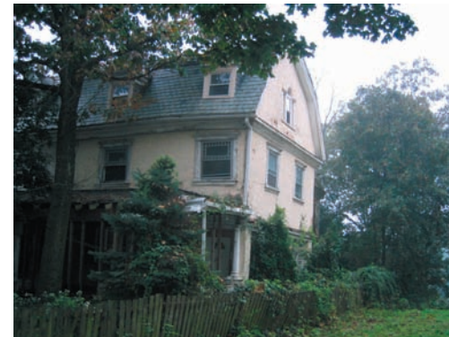
Example of a large deteriorated house.
