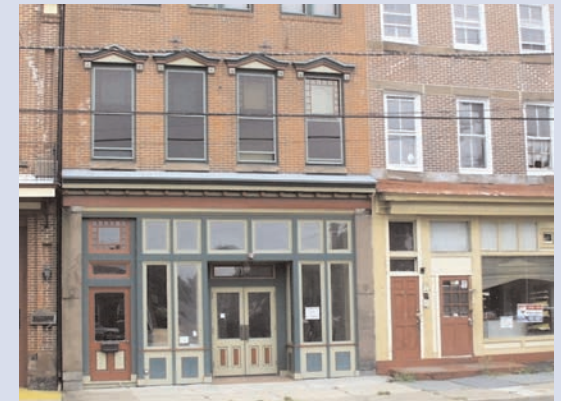
Empty storefronts on East Broad Street.
