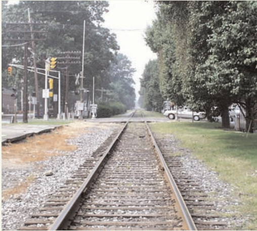
Existing rail line, Palmyra.
