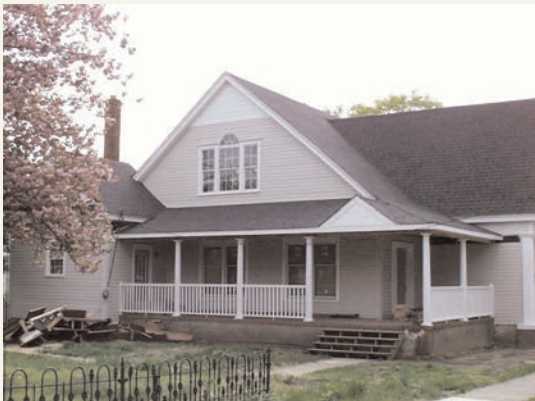
Infill housing near central business district.
