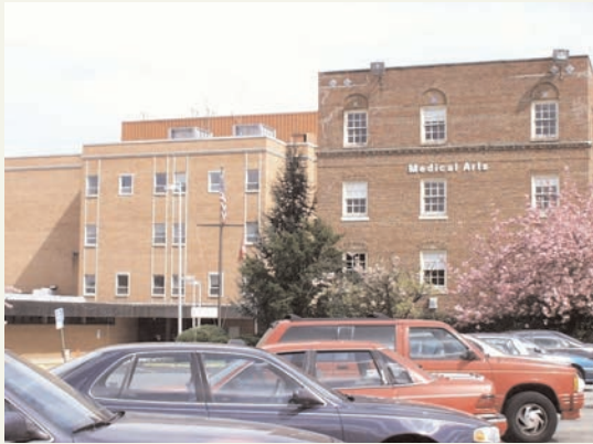
Zurbugg Hospital, with age - restricted and assisted living residential units.
