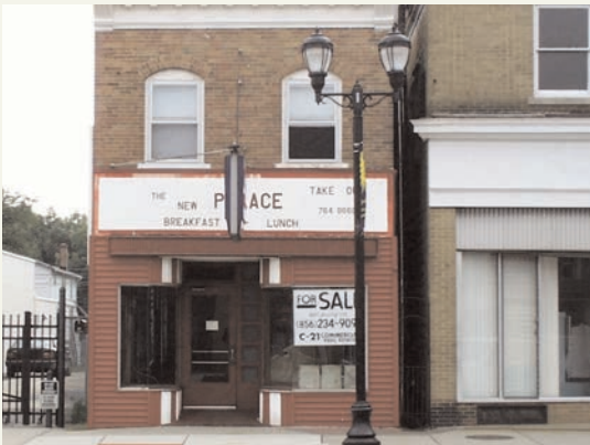
Empty Storefront on Scott Street.
