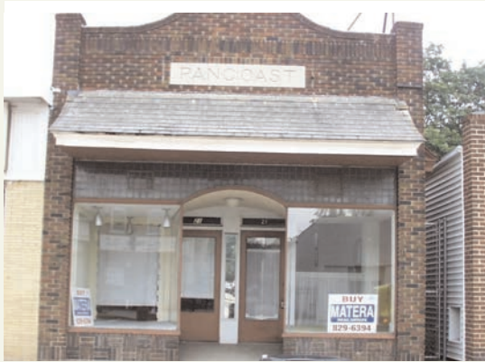
Empty storefront on Scott Street.
