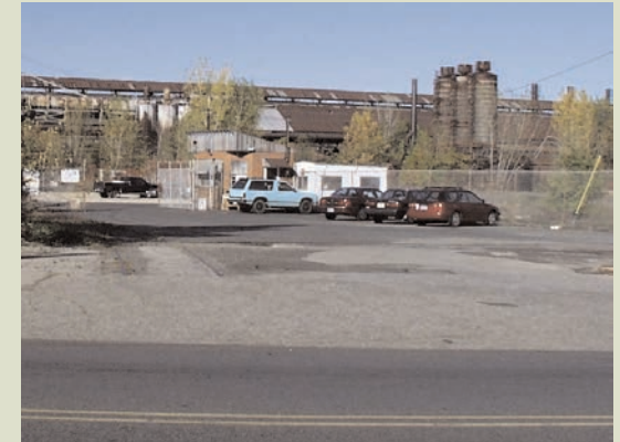
Access from Hornberger Avenue to future station site.
