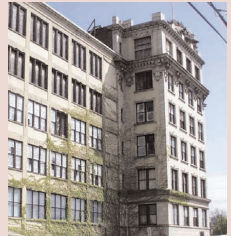
Riverside's Watchcase Tower presents a potential market for condominiums and apartments, some age - restricted units.
