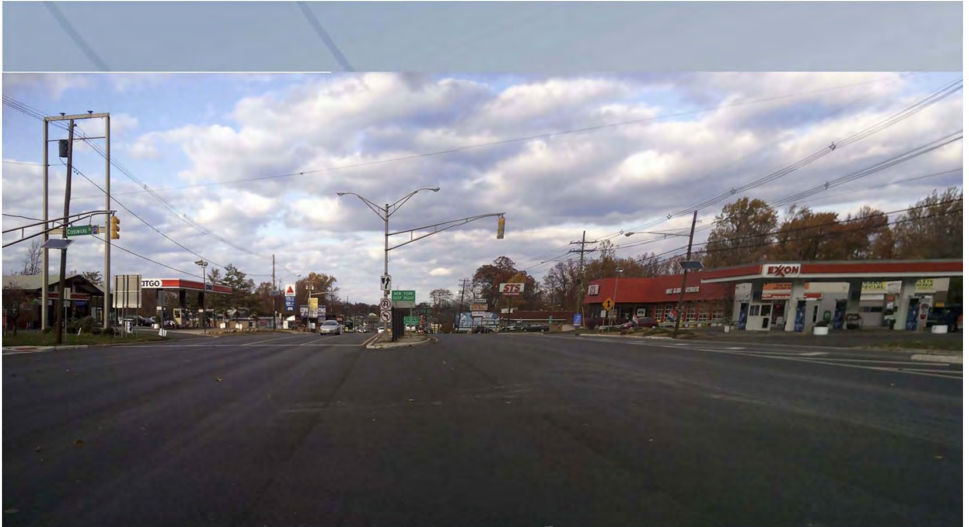
Existing: Northbound View of Route 130/206
