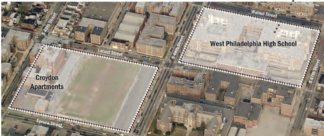
West Philadelphia High School and Croydon Apartments
