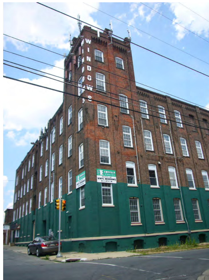
Industrial building near Temple Regional Rail Station
