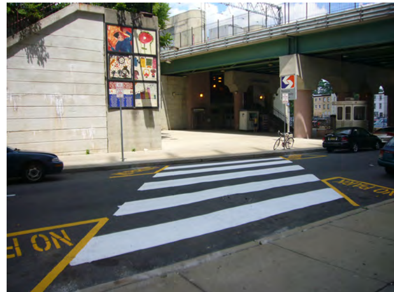
Existing Temple Regional Rail Station Plaza
