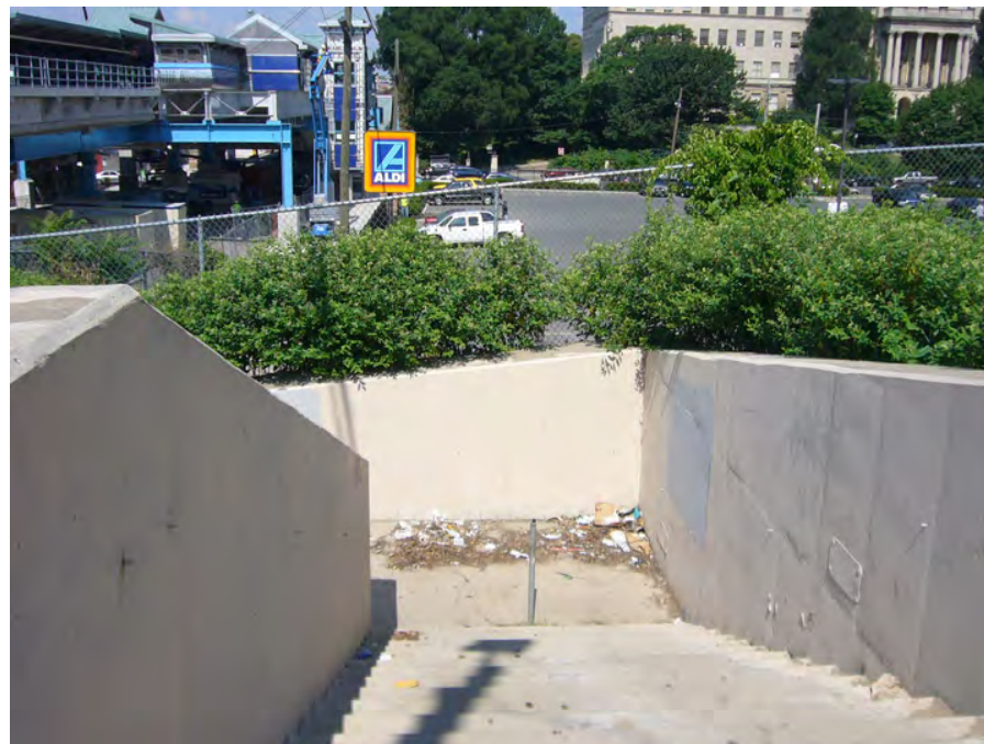
Westpark Apartments staircase
