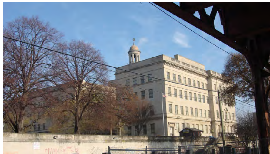
Provident Mutual building (4601 Market Street) next to 46th Street Station
