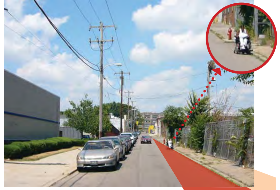
Narrow sidewalk on Ludlow Street
