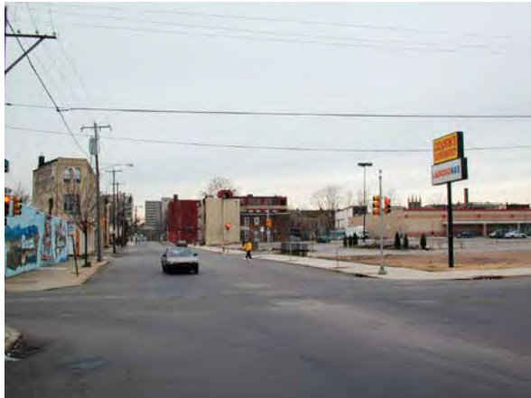
6th and Berks Top: Existing intersection Top right: Street section showing existing cross-section Bottom right: Proposed travel lane reduction, median, colored bike lane and landscape buffers
