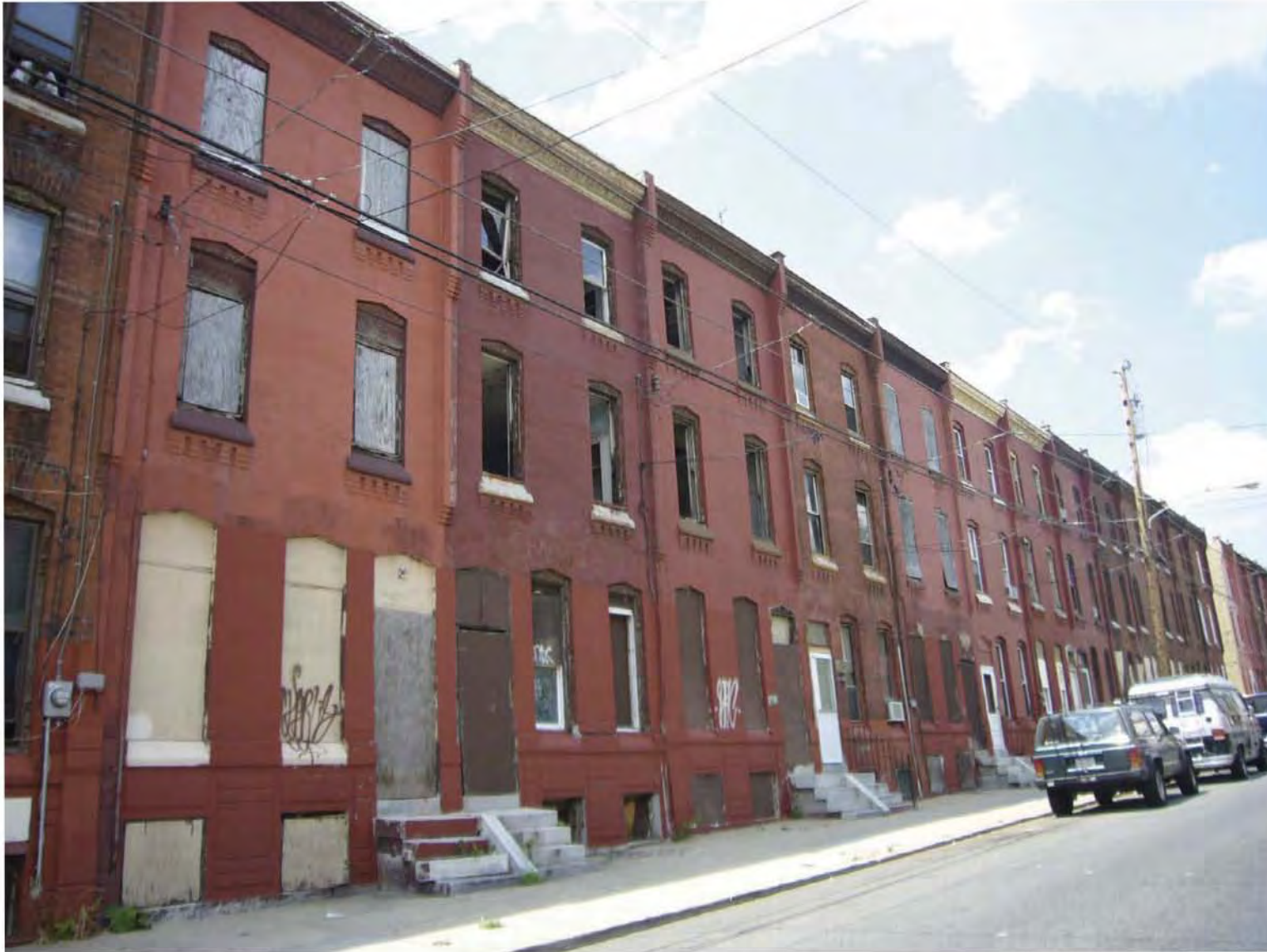
Houses in need of rehabilitation along 9th Street
