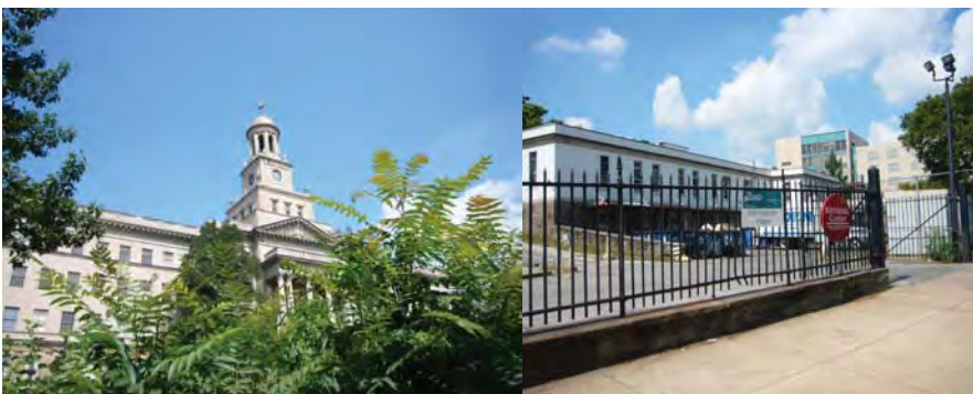
46th Street Station Area (L-R): 4601 Market, Kirkbride Center
