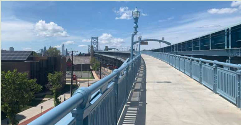
The bike ramp on the Ben Franklin Bridge received $3.8 million in Transportation Alternatives Program funding
