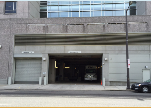
Off-street loading at the American College of Physicians Building
