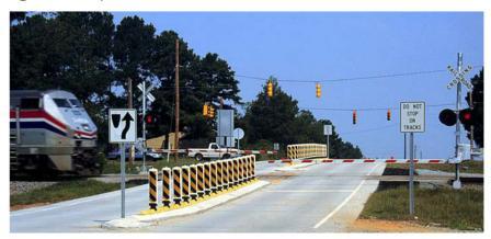
Figure 12: Example of Mountable Raised Curb Channelization Device
