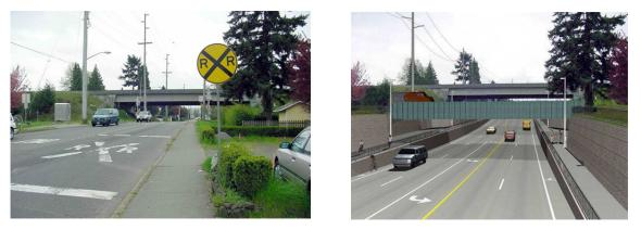
Left: Present at-grade conditions at M Street in Auburn, WA. Right: A rendering of a planned roadway tunnel under the rail line in Auburn, WA. (Source: Puget Sound Regional Council)
