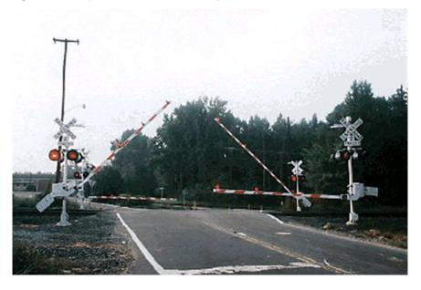
Left: A four-quadrant gate in North Carolina (note: the gates to the entrances are already closed, but the gates for the exits are in the process of closing). (Source: North Carolina Department of Transportation)
