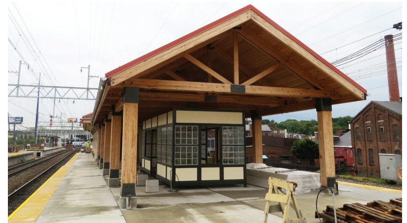
TIP projects often include elements that are not immediately visible. SEPTA's Wayne Junction Station, above, was replaced and upgraded. At the same time, the traction power supply system for SEPTA's regional rail service was upgraded in this location.
